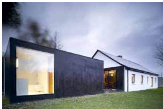
Figure 16.49 Extension to side of house. Glengowla, Co. Galway. Boyer Kennihan Architects.
