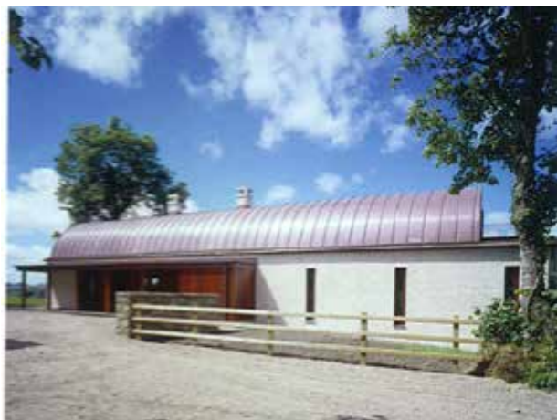
Figure 16.29 Barrel Roof, Rosslea, Co. Fermanagh. Aughey O'Flaherty Architects.
