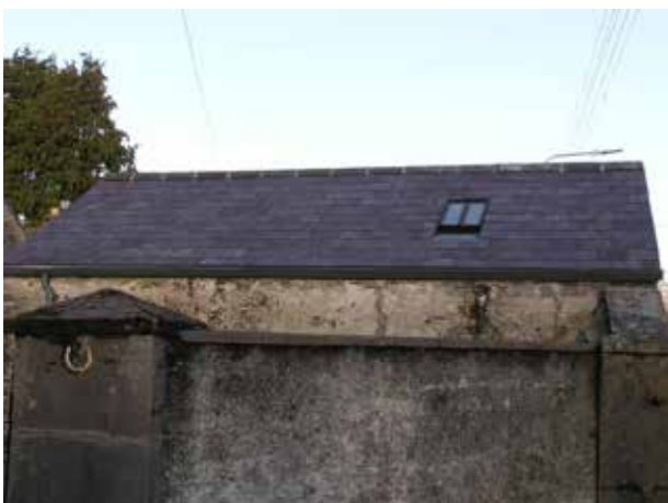
Figure 16.30 Example of traditional rooflight flush with slate detail; Naas, Co. Kildare
