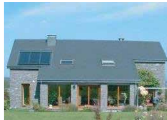
Figure 16.46 Image of roof solar panel
