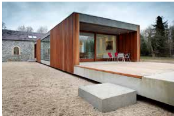
Figure 16.47 Refurbishment and Extension. Ballymahon House. ODOS Architects.
