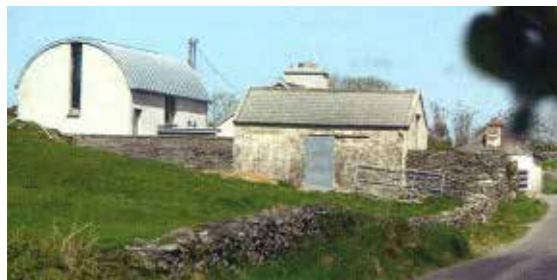
Figure 16.48 Cottage Renovation and 'Barn' Roofed Extension. Michael Kelly Architects.
