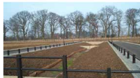
Figure 15.13 Swales at Upton, Northhampton, UK
